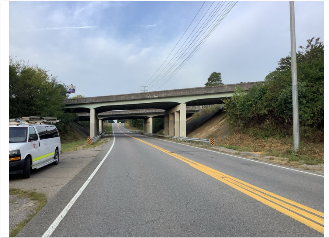
Elevation right and underpass forward
