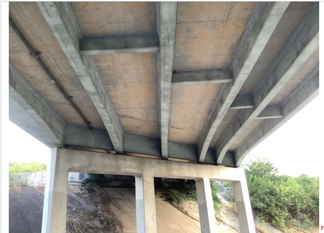
From bent 1 - view underneath
