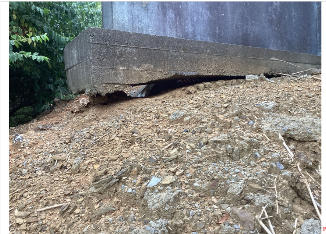
Wing 1 right - Undermining 8' long
